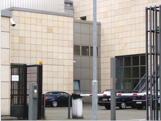
Vehicle access control
