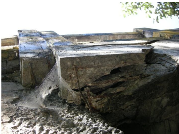
Photo 15.17: Dilapidated Condition of Ranipool Bridge
