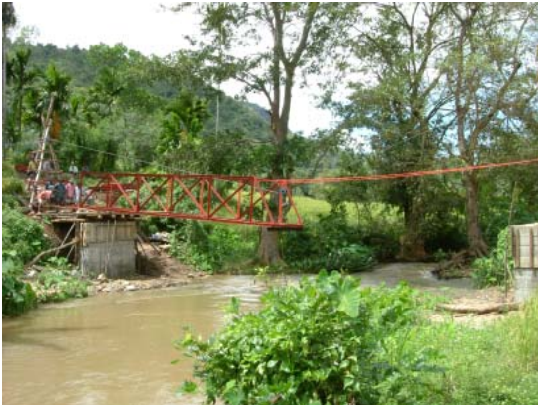
Figure 7.15: Use of Cable Trolley to Install a Modular Steel Truss Footbridge
