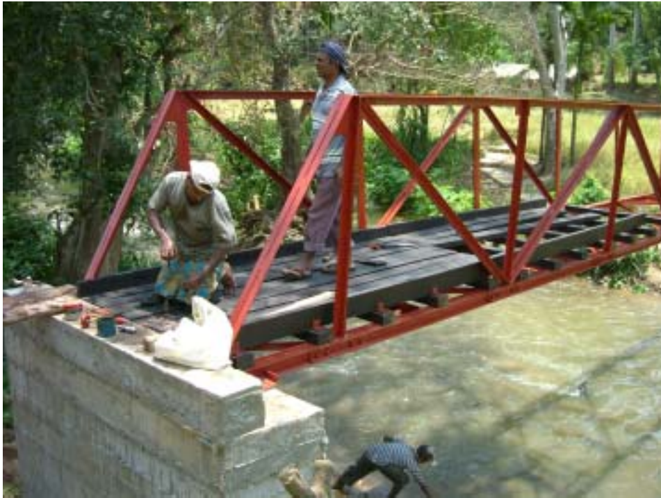
Details of construction and attachment of decking
