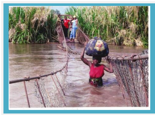
Villagers crossing a broken bridge in rural Southern Tanzania
