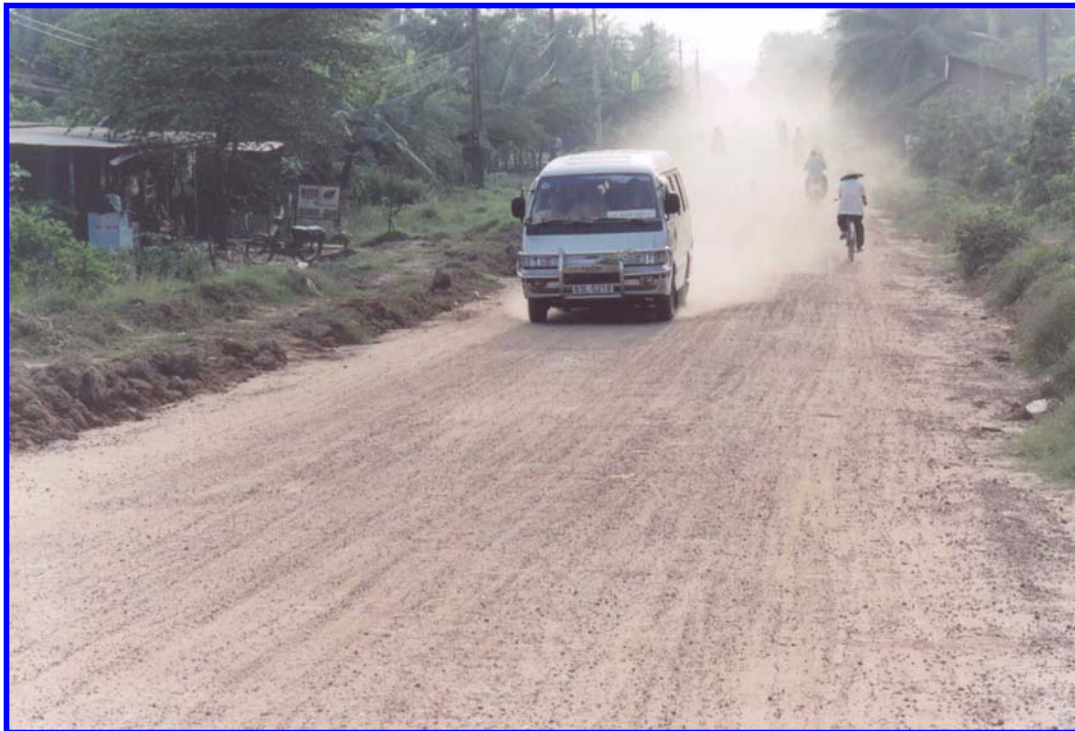
Photographs VIII : Dust emissions & material loss in dry weather
