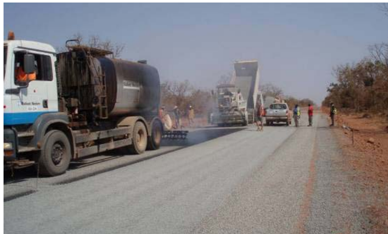
Figure 34: Application of chippings immediately after the application of binder
