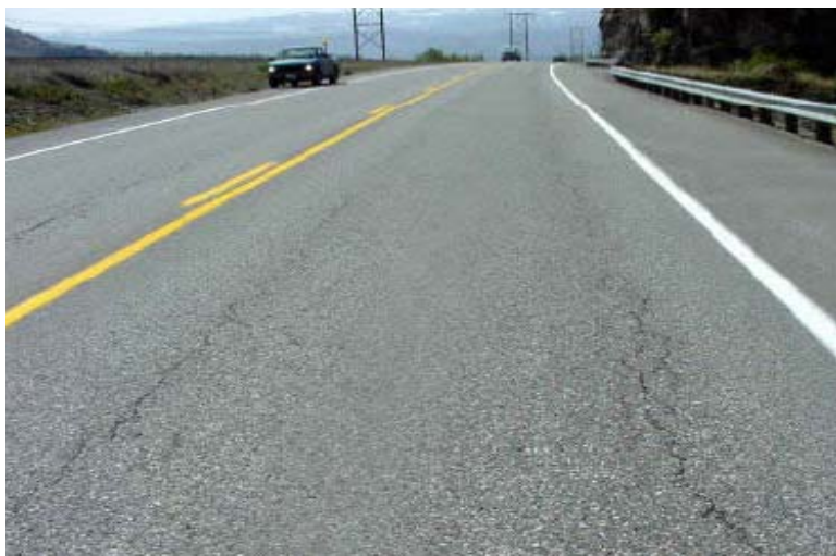
Figure 65: Longitudinal cracking
