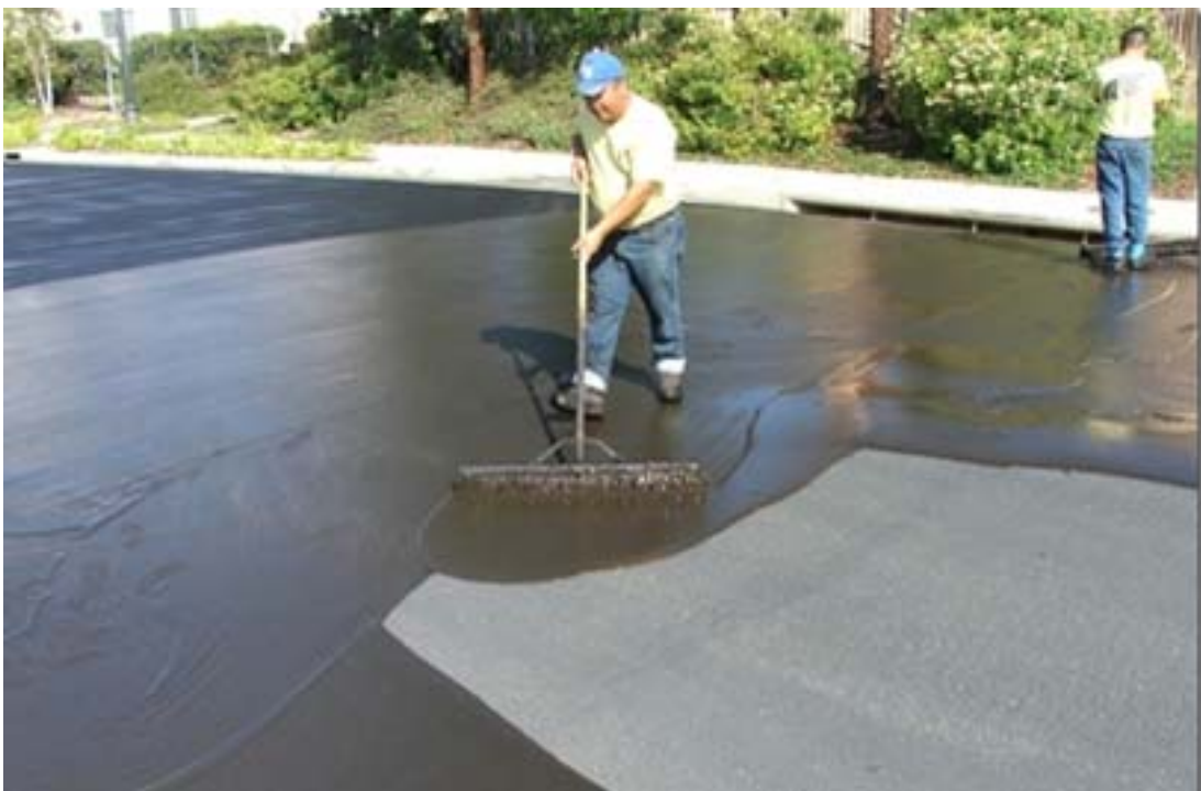
Frame No: 010 Description: Spreading Slurry by Squeegee (United)
