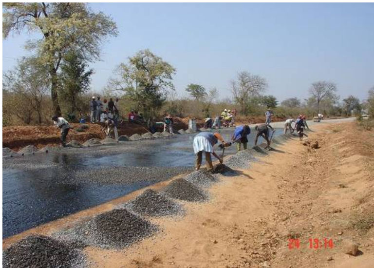
Figure 37: Spreading of aggregates by hand
