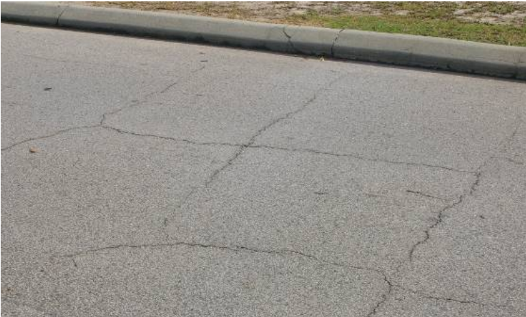
Figure 68: Block cracking
