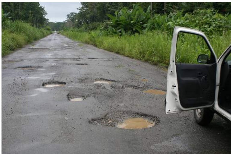
Figure 60: Potholes
