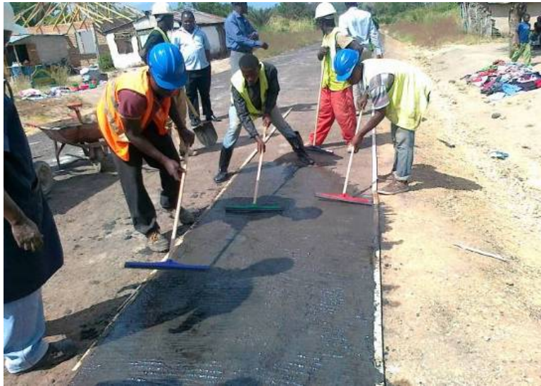
Figure 42: Spreading the slurry using squeegees
