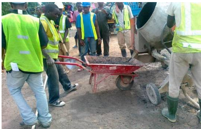
Figure 41: Transporting the slurry to the location of application
