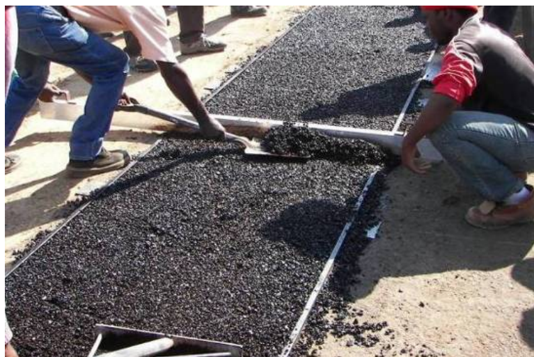
Figure 48: Placing the cold mix asphalt by spade
