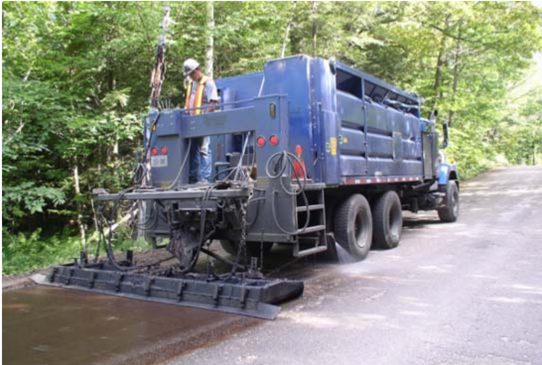
Frame No: 009 Description: Slurry Seal Machine (Duncor)
