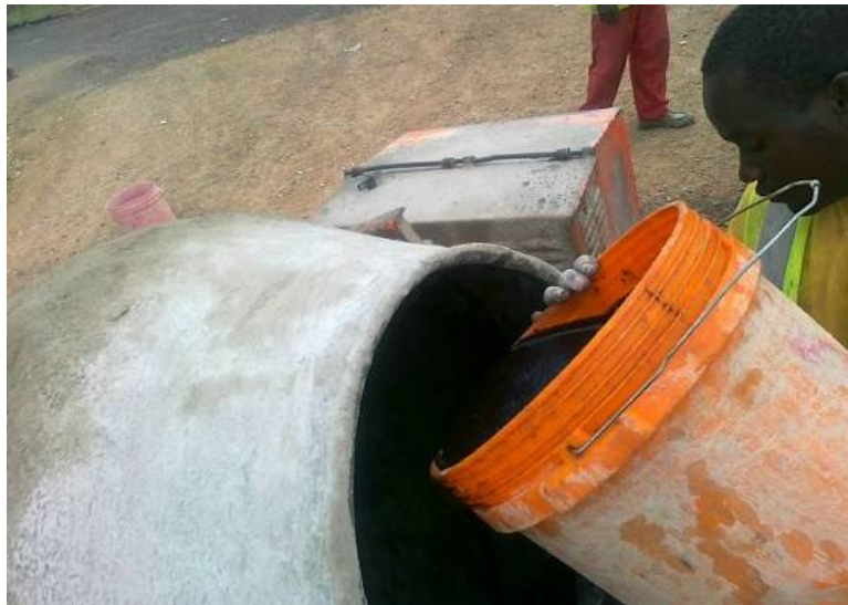
Figure 41: Transporting the slurry to the location of application
