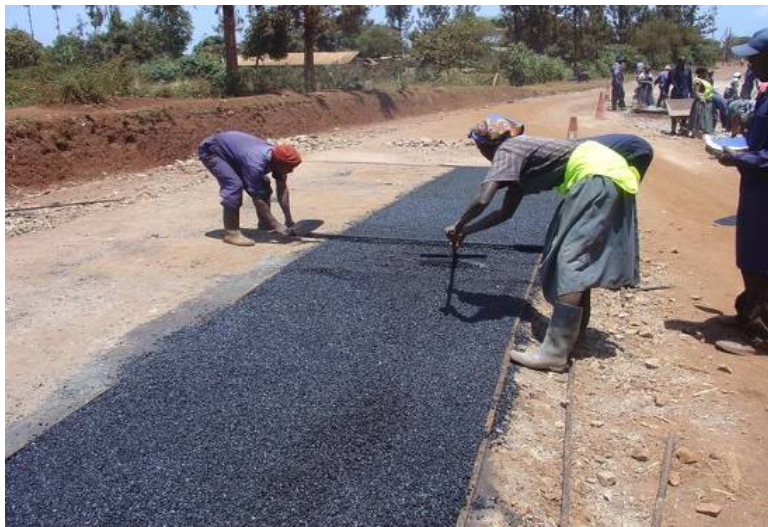
Figure 49: Levelling the cold mix asphalt
