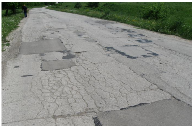
Figure 57: Defective patching
