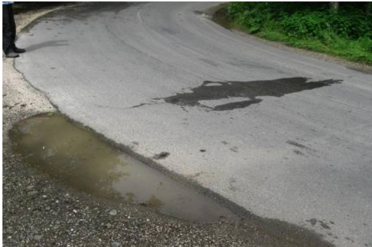
Figure 63: Poor drainage
