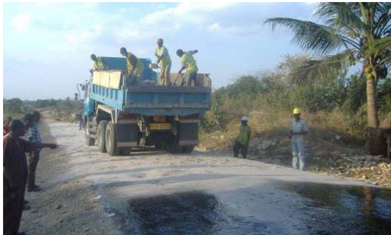
Figure 39: Construction of a sand seal
