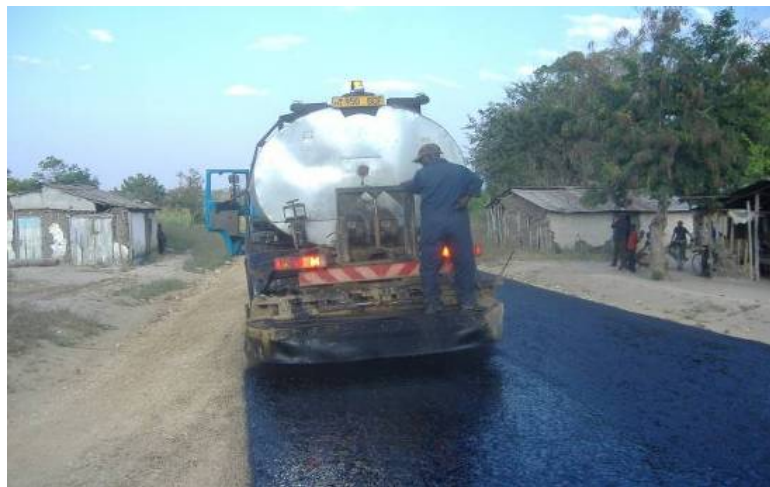
Figure 33: Application of a prime coat
