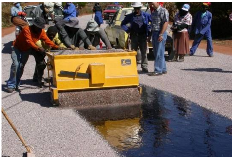
Figure 38: Spreading aggregates with a Chippie
