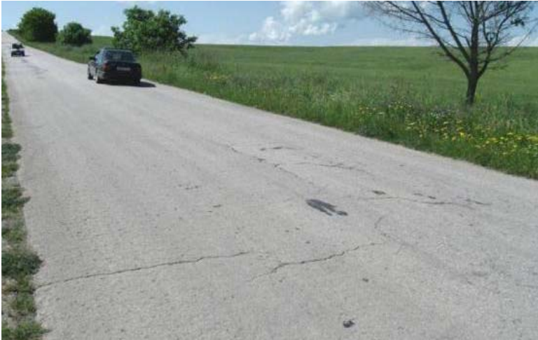
Figure 66: Transverse cracking
