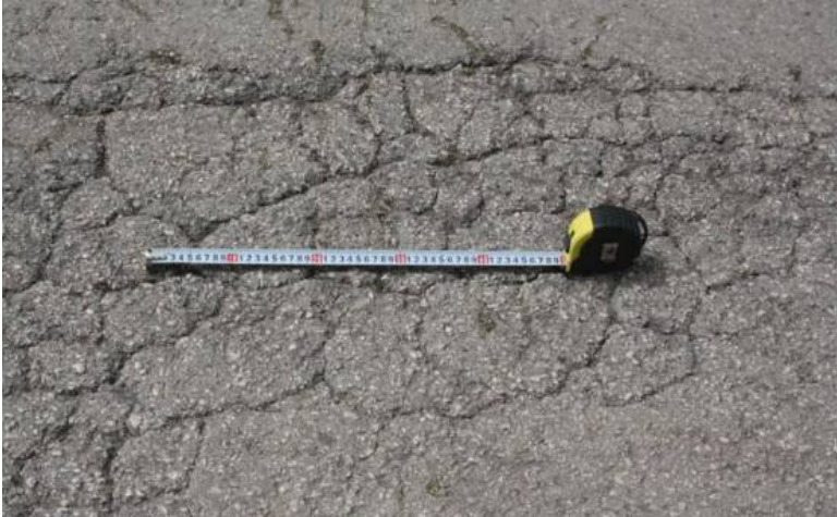
Figure 67: Crocodile cracking
