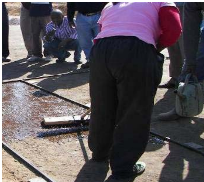
Figure 44: Spreading emulsion
