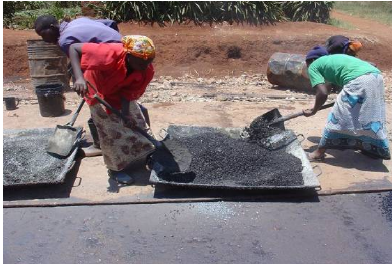
Figure 47: Mixing cold mix asphalt
