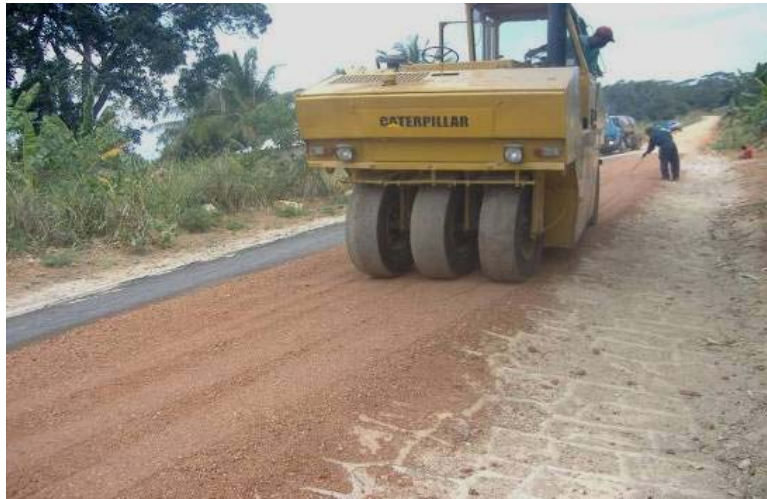
Figure 35: Rolling an Otta seal
