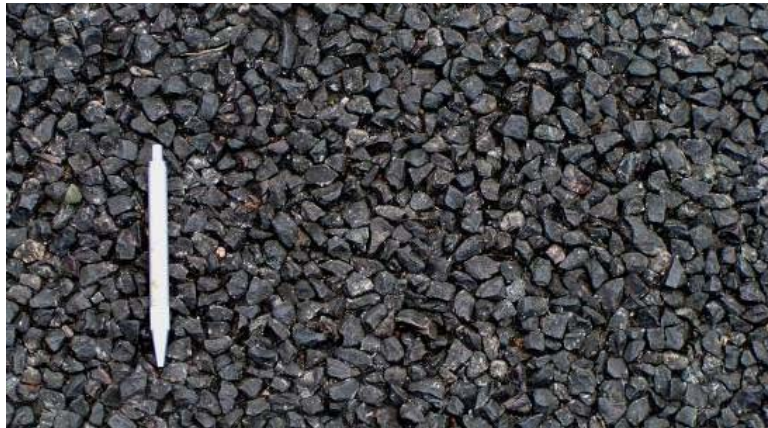
Figure 54: Fog spray applied to a single surface dressing
