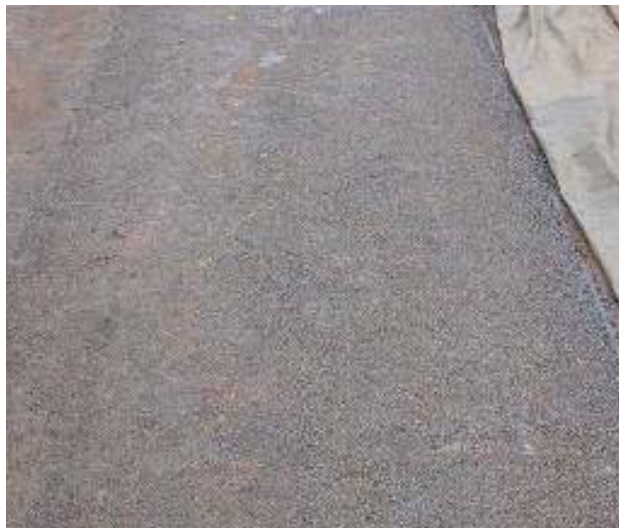
Figure 53: A well constructed joint
