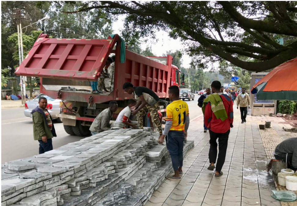
Figure 36. Footpath construction in Addis Ababa.
