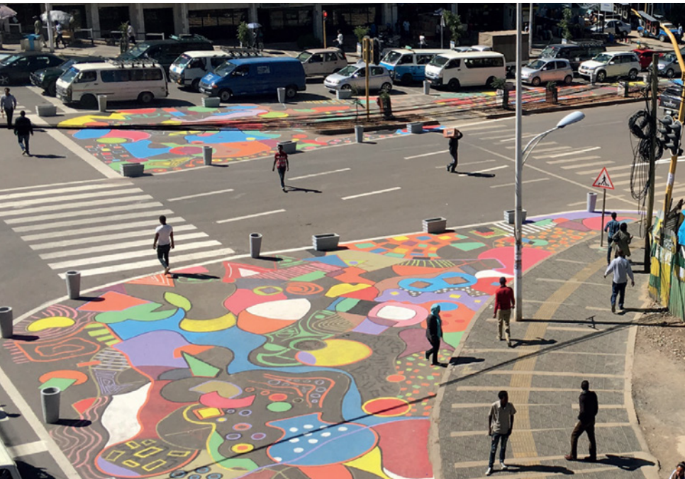
Figure 24. Intersection modifications in Addis Ababa have reduced lane widths and turning radii for motor vehicles in order to improve pedestrian safety.
