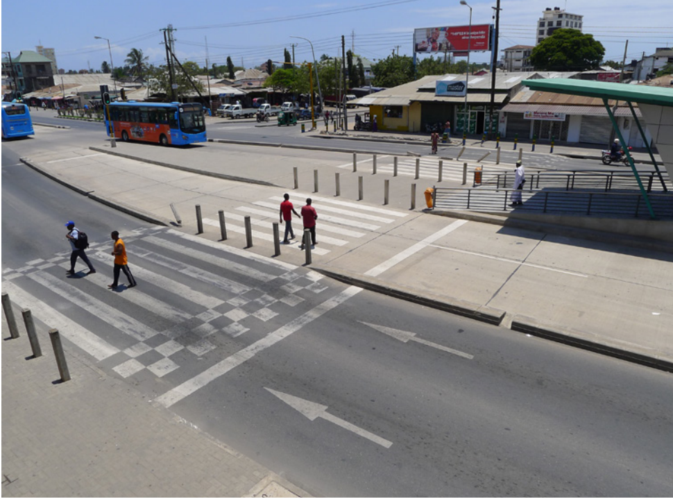
Figure 20. Table-top crossings reduce the speed of motor vehicles and ensure universal access for pedestrians.
