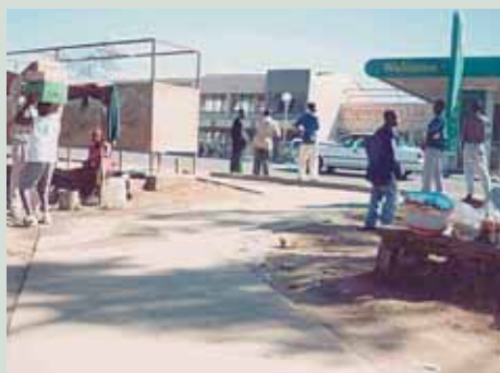
Figure 3.5 A new paved pedestrian footway is provided to ensure access for pedestrians and wheelchair users to the minibus stop. A new bus shelter, that is fully accessible to all users is under construction at the same site.
