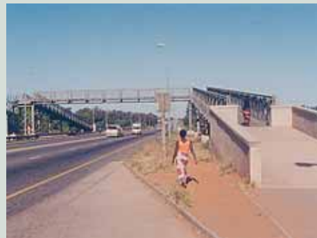
Figure 2.11 A pedestrian bridge enhances safety over this busy national road in Mozambique
