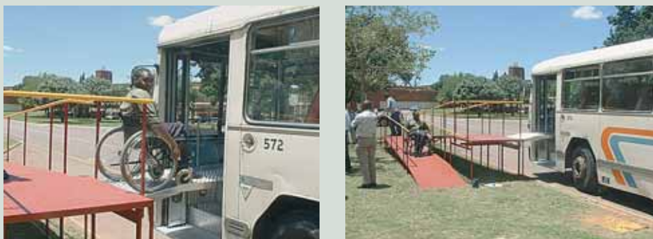
Figure 3.31 Illustrations of bus wayside platforms, Pretoria, South Africa
