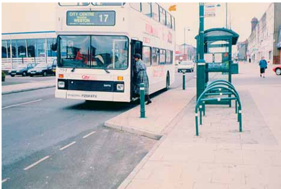
Figure 3.24 A bus bulb or boarder in operation
