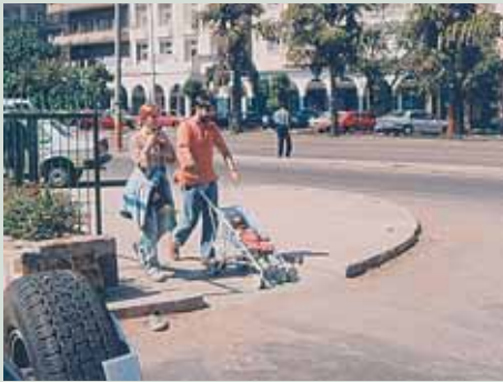
Figure 2.9 Provision of kerb ramps benefit all users
