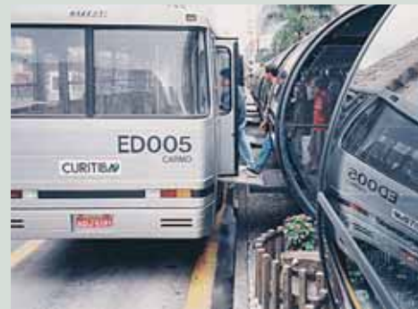
Figure 3.28 Raised bus tubes from which passengers board at floor level into buses (such as in Curitiba, Brazil) (Photo by Charles Wright)
