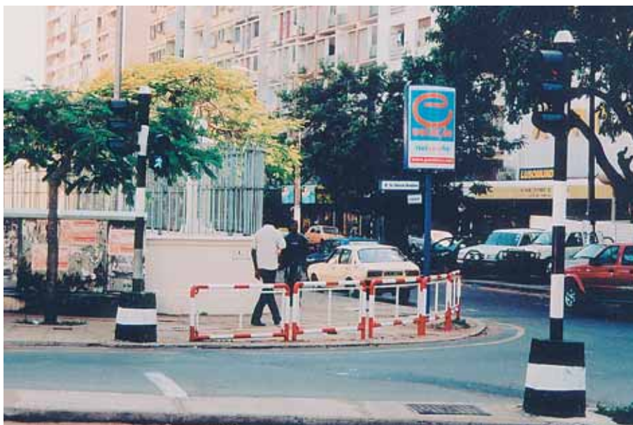
Figure 3.3 Physical barriers such as guardrails may help to improve the safety of vulnerable users in dangerous situations such as busy street crossings
