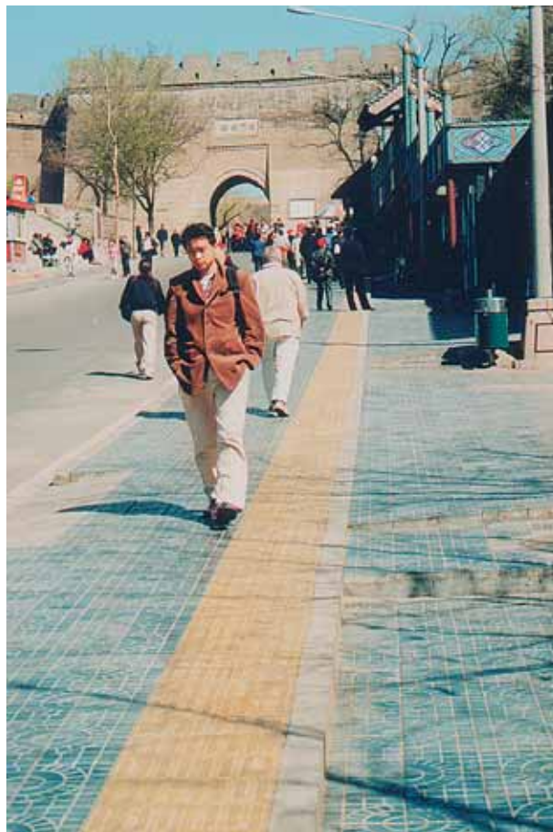
Figure 3.15 Tactile guideway with colour contrast in use in China
