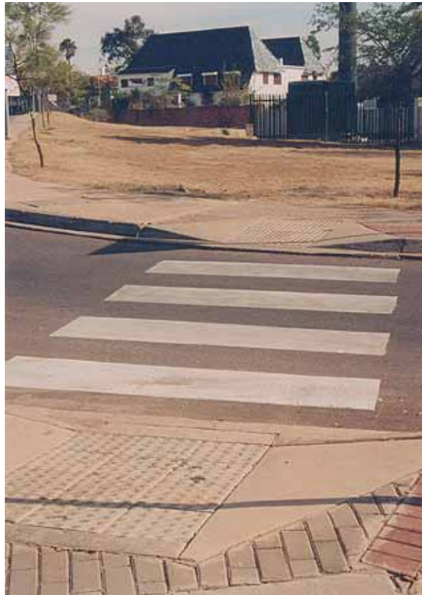
Figure 3.16 Tactile warnings on kerb ramps used in South Africa
