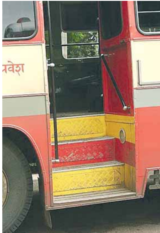
Figure 3.42 Low-cost improvements to this bus entrance included installing extra handrails, colour contrasted steps and lighting
