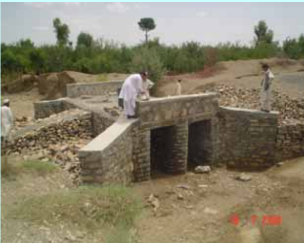
Ongoing work for Culvert construction
