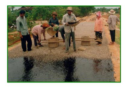
A range of surface and paving options is available using bitumen as a seal or binding material. They can be particularly suitable for labour based methods if emulsions are used. Techniques include 'chip' seals, sand seals, gravel seals, and bitumen macadams. The thin seals will require suitable pavement layers to be constructed between the road foundation and surface.
