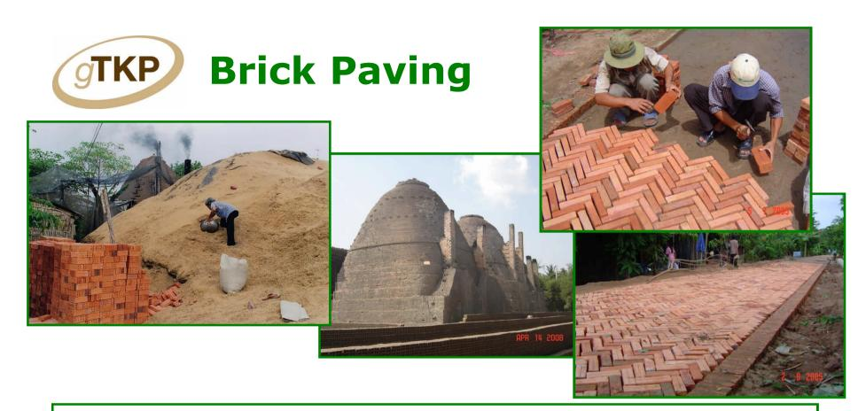
Burnt Clay Brick paving can be an important option in areas lacking hard stone resources, for example in delta regions. The clay can be fired to high quality bricks using small scale kilns and renewable energy sources, such as waste rice husk. Materials haulage can be minimized and local employment created in brick production for roads and building construction.
