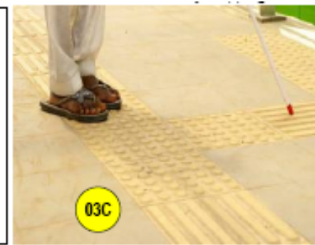
Engineering configuration of floor tactile tiles
