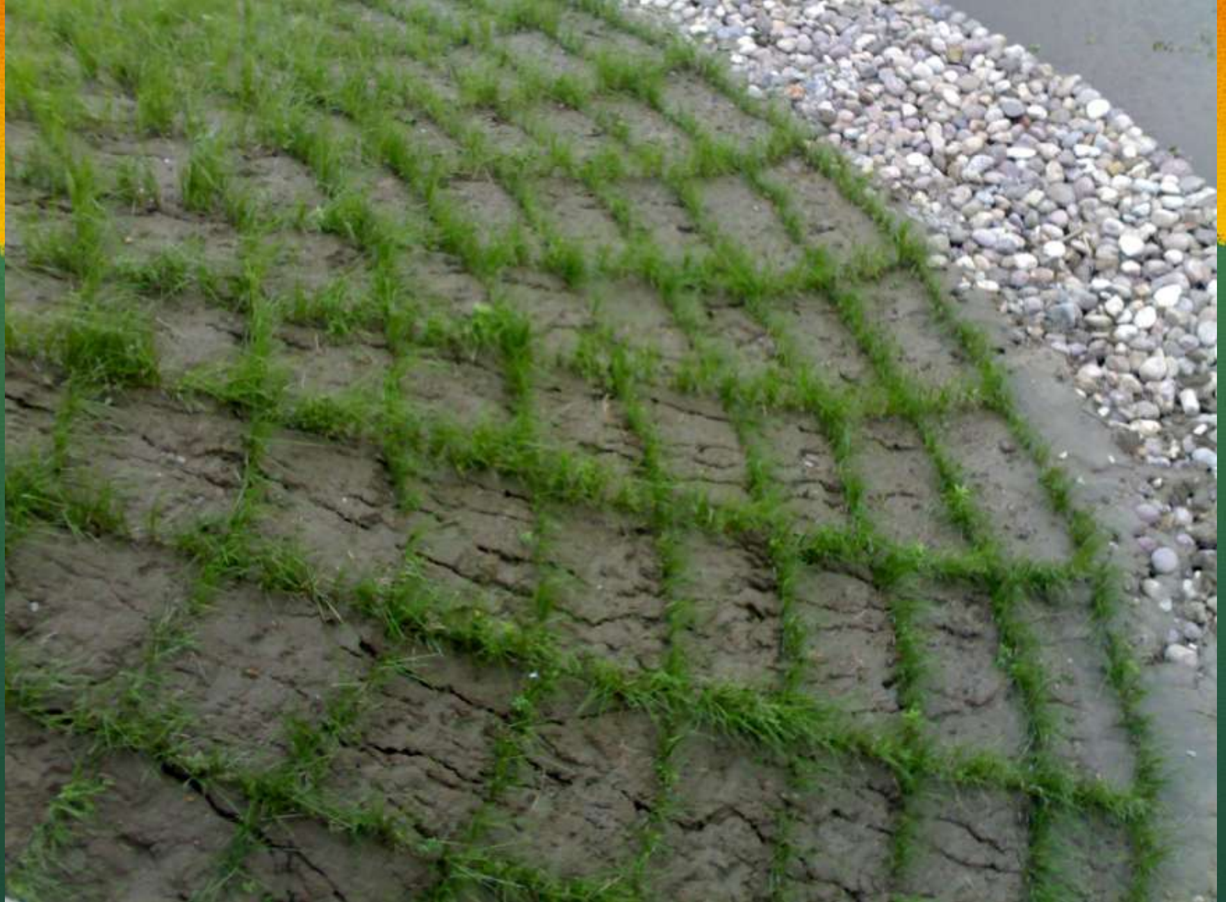
The forward slope with toe protection
