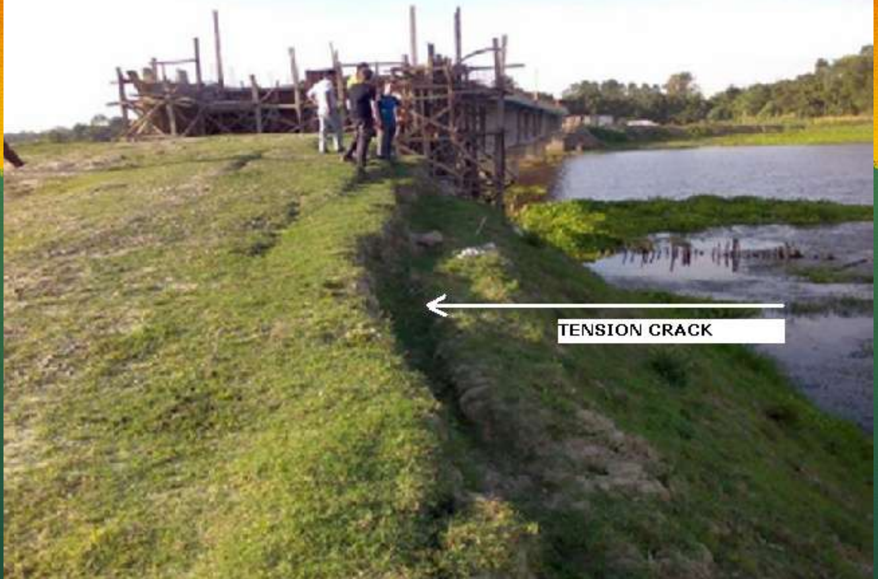
Doria bridge approach in Majuli; during construction
