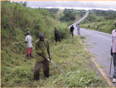
Grass cutting—a typical, labour-based routine maintenance activity.
