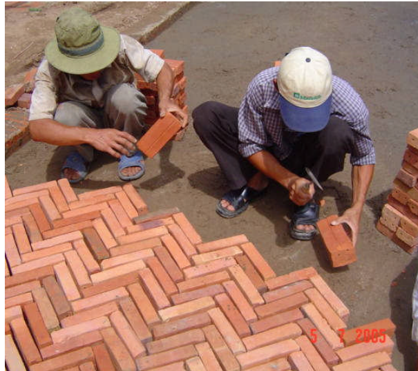
Photo 7-2: Example of burnt Clay Brick surfacing
