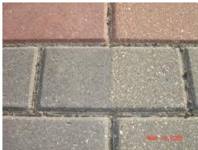
Photo 7-3: Example of concrete brick paving (Stretcher pattern)
