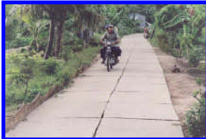
Photo 7-5: Example of concrete surfacing
