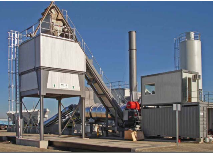
Figure 5: ContiMix asphalt plant
