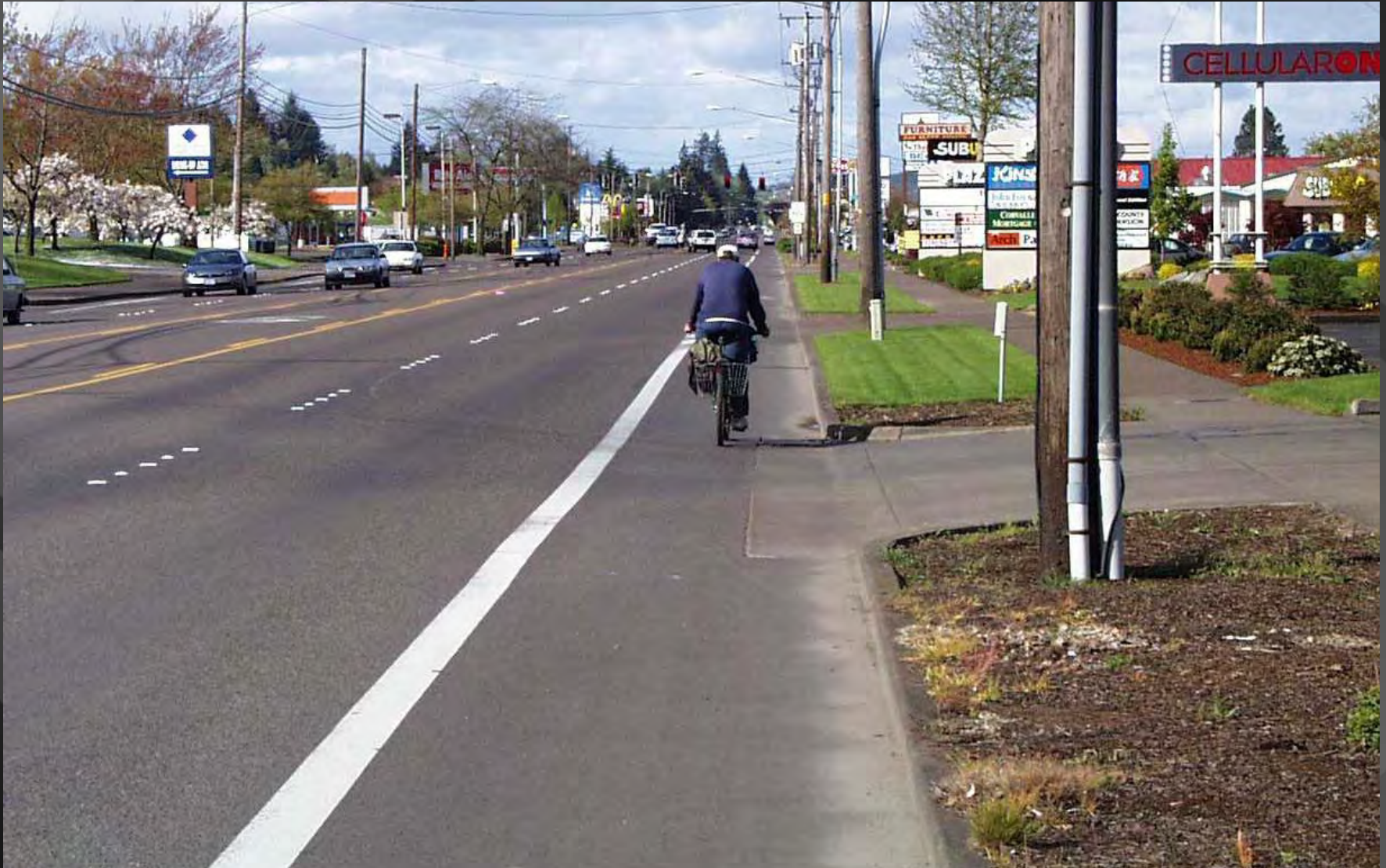
A commercial arterial w/ bike lanes & sidewalks
