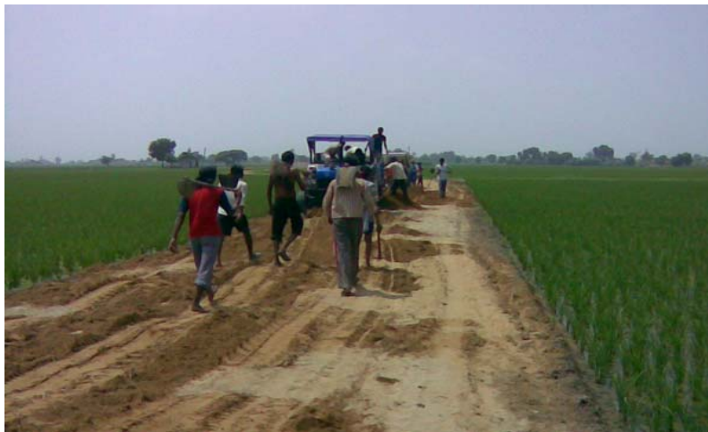
Photo 2 – Earth works being done by Villagers
