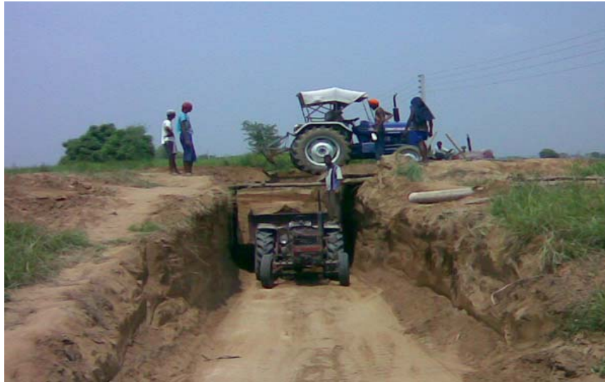
Photo 3 – Innovative approach to load earth using common agricultural machinery
