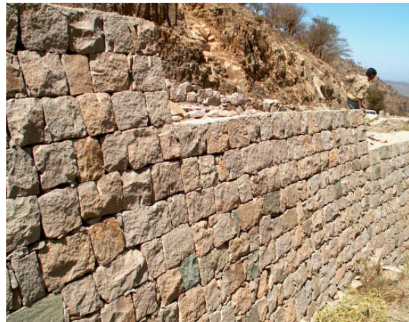
dry stone masonry retaining wall
