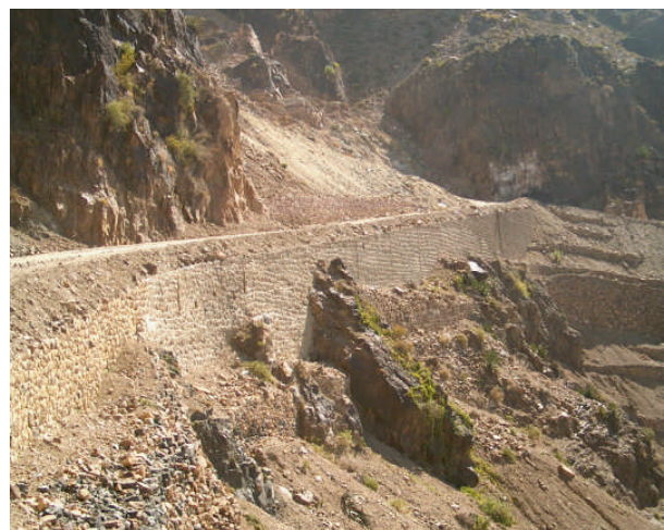
long and high retaining wall
