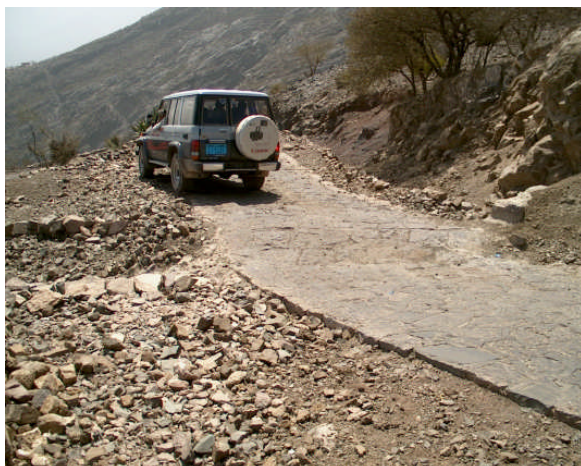
drift as cross drainage
