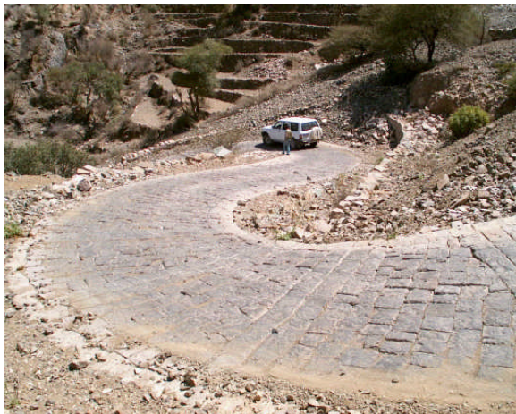
hairpin bends with stone paved surface
