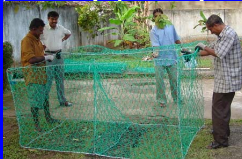
Tying panels together to complete gabion basket
