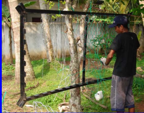
Locally fabricated gabion weaving frame
