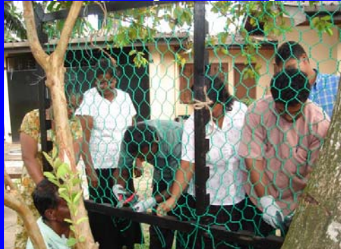
Community members during on site practical training in gabion weaving
