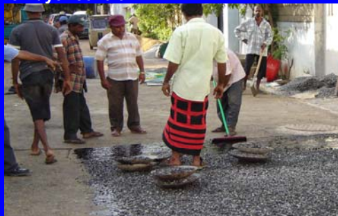
Sealing works using bitumen emulsion
