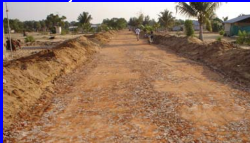
Completed section of compacted sub-base
