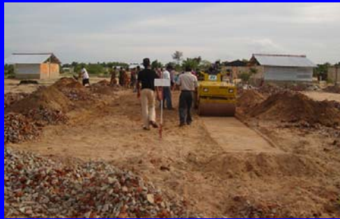
Excavation of Subgrade for sub-base placement
