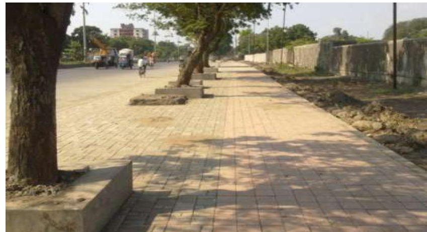
Trees retained along Footpath
