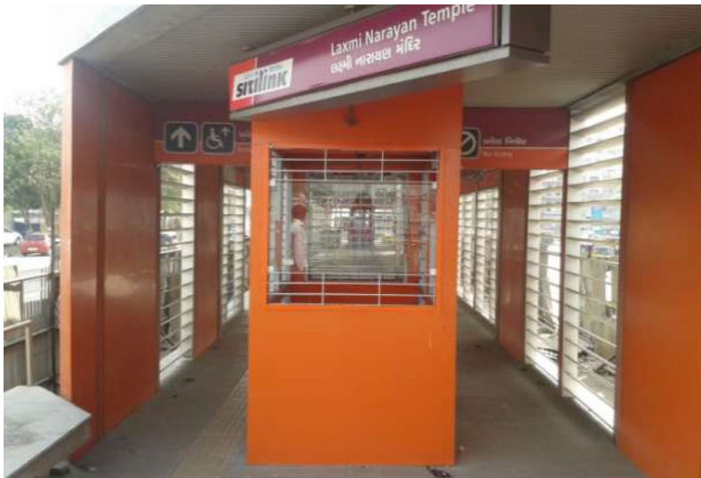
Prototype Bus Station Completed
