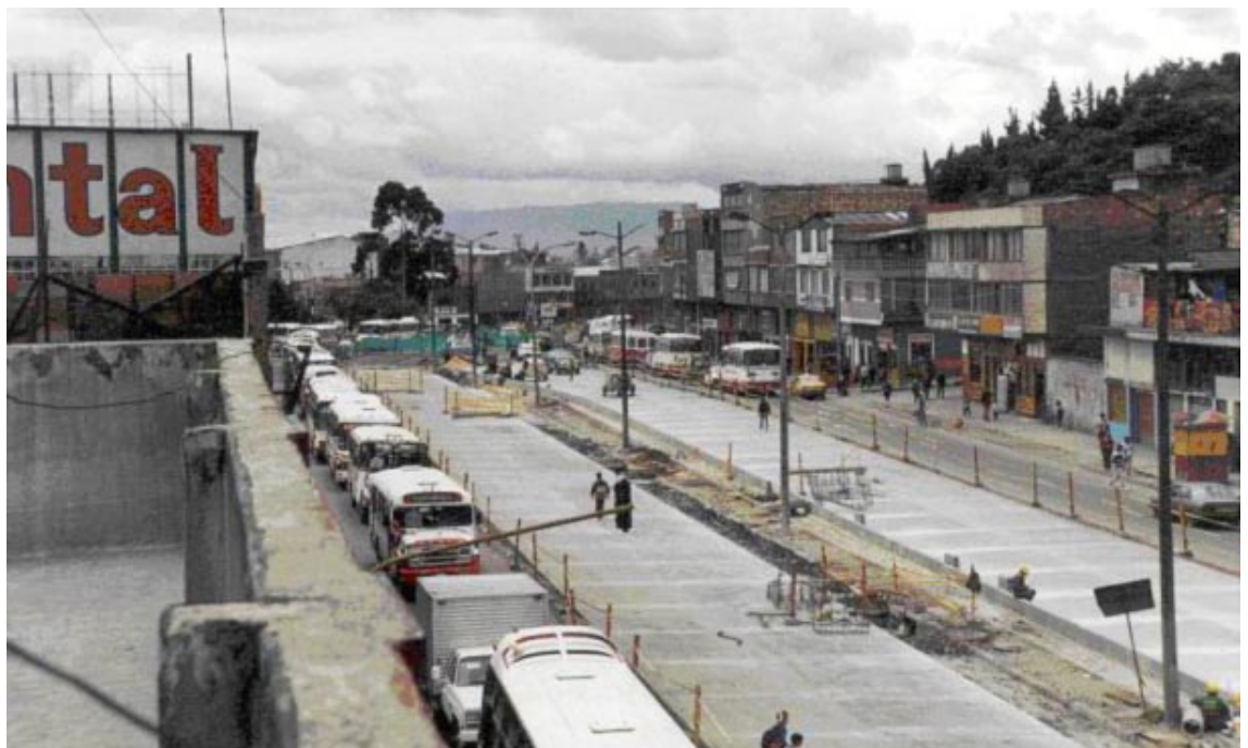
Fig. 20.33 The disruption to traffic and businesses during Phase I construction of TransMilenio did receive some criticism. More mitigation measures were subsequently applied in Phase II.
