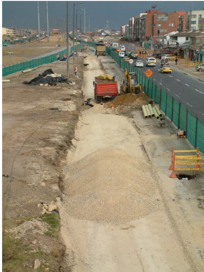
Fig. 20.29 Construction on the Americas corridor in Bogotá.
