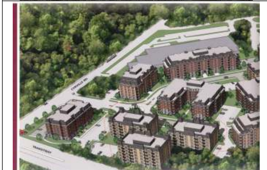
Place de Gouverneurs site with the first three buildings and the full Site Plan showing site access to the Transitway (courtesy Richcraft)
