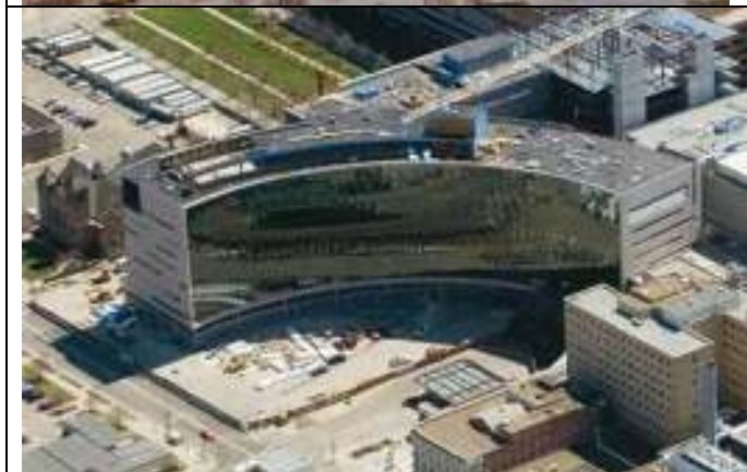
On top, the parking garage that occupied the site of the new Cleveland Clinic Heart Center. Below, the state of construction as of July 2007. The promenade in front of the center will provide direct access to the BRT.
