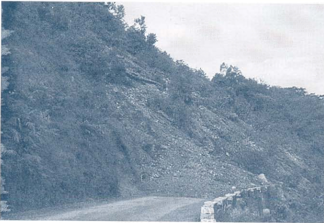
Shallow planar failures on long steep slopes can give rise to large volumes of debris. Although the debris in this example is about 5m deep, the depth of the failure itself is less than 1m
