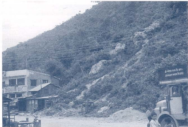
The road at Anboo-Khaireni crosses the base of a semi-stable colluvial slope
