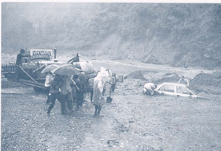
Liquefied debris from a large landslide is deposited wherever the gradient allows. In this case, the natural deposition site was the point at which the road crossed the month of the valley
