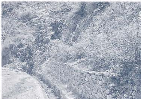
Shrubs planted above a toe wall catch loose debris moving down the slope
