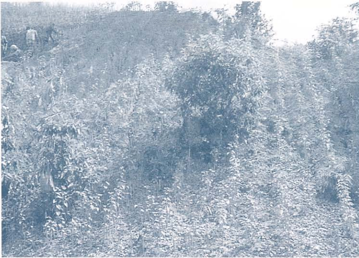
Downslope planting lines allow rapid surface drainage of this impermeable Siwalik mudstone, while still armouring the surface against erosion
