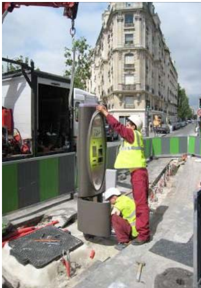
Figure 11 - Construction of a Vélib station in Paris
