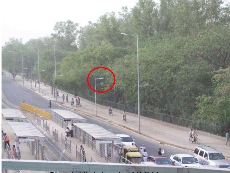
Special lighting for NMT lanes
