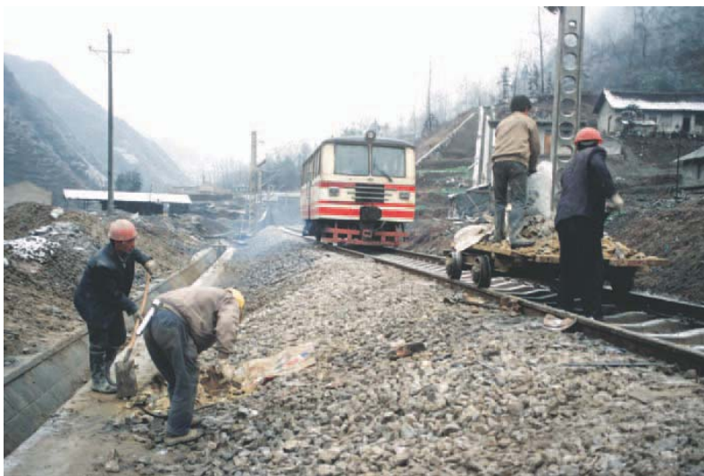
Throughout the country, railway construction generates substantial direct and indirect employment.
