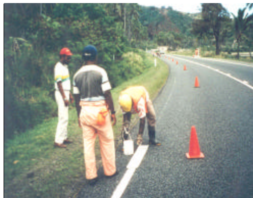
Plate 1 (left): Road marking to improve safety.
