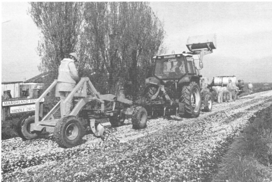
Figure 16 - Tractor with Loader, Harrow and Light Towed Grader for Bitumen Road Rehabilitation
