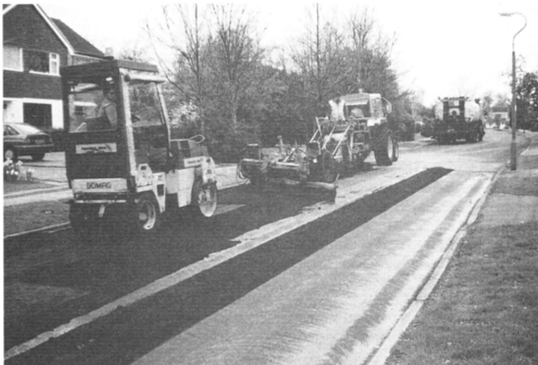
Figure 5 - Bituminous Overlay Using Tractor Towed Asphalt Spreader
