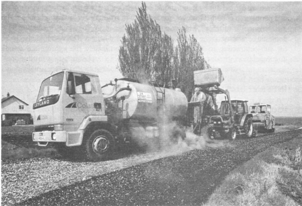
Figure 4 - Bitumen Pavement Reconstruction Using Tractor Harrow
