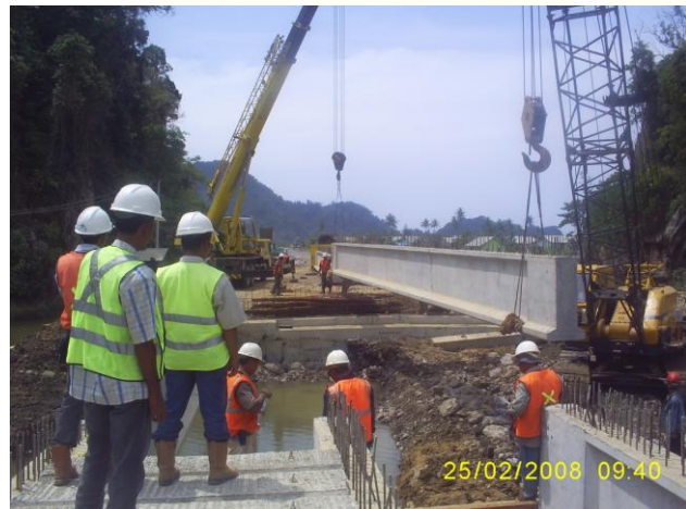
Inspectors monitor erection of a girder at Kalla Bridge (Km 45+240 – Section 3
