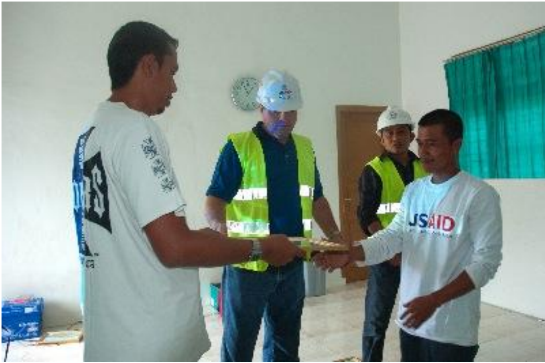
After the 10-hour course, participants were given certificates confirming they had completed basic level construction safety training.
