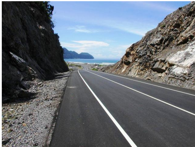
The Indian Ocean looms beyond a large rock cut section of the Aceh Road corridor.
