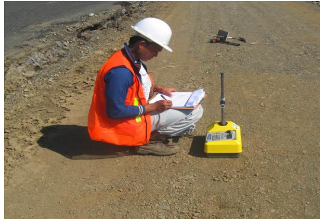
An engineer examines the embankment's density using a nuclear densitometer.
