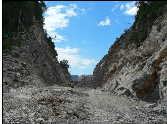
The Saddle has been breached. The road will soon be constructed.
