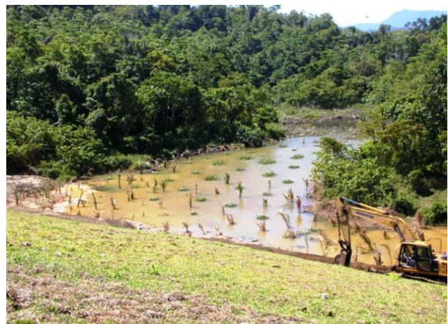
Measures were taken to mitigate the impact of the road construction on the environment. Curtains were installed at bridge and culvert sites to prevent sedimentation into the waterways. A wetland was created at the base of a high embankment area by planting Nypah palms, Giant leather ferns, Phragmites (reeds) and floating native species.
