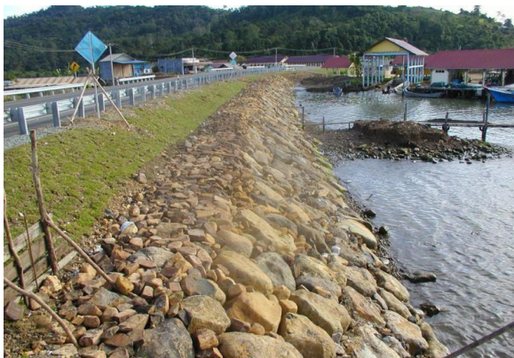
Embankment slopes along the coastline are armored to endure storm surges.
