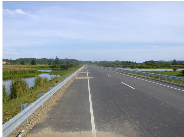
Before / After of construction of new corridor through swamps to provide a more direct and safer alignment. Geotextile was employed to minimize differential settlement.
