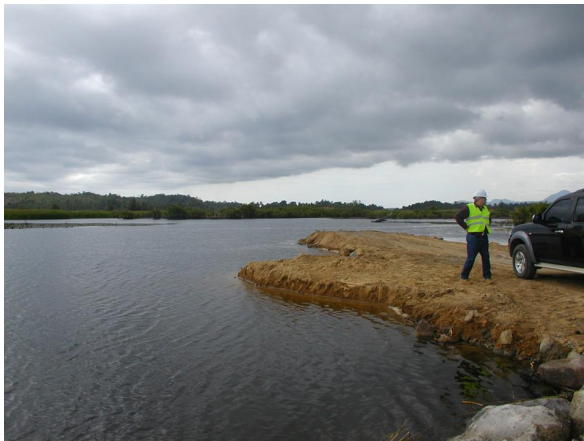
Before / After of construction of new corridor through swamps to provide a more direct and safer alignment. Geotextile was employed to minimize differential settlement.
