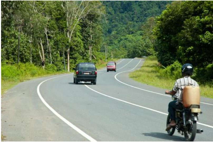
The new Aceh Road between Banda Aceh – Lamno
