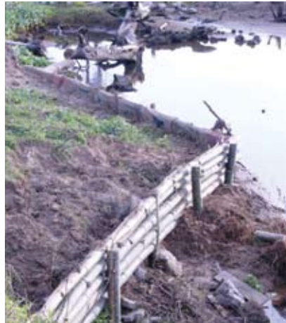
Silt traps at the Raba River Bridge Penangkap sedimen di Jembatan Krueng Raba
