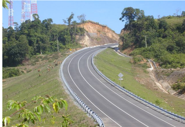
Use of large cuts and high fills to construct the new road in its most direct alignment enables faster travel using less fuel and with less wear and tear on vehicles, which results in a greater boost to the economy with a smaller impact on the environment.
