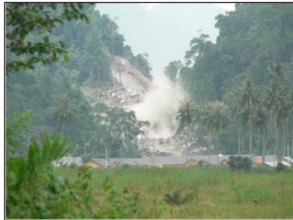
The rock at Pudeng Saddle is hard. Blasting is required.
