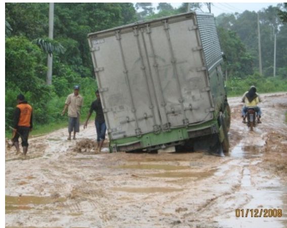
The emergency road constructed by the Indonesian military immediately after the tsunami was a source of dust on the villages during the dry season and was muddy and often impassible during the rainy season.
