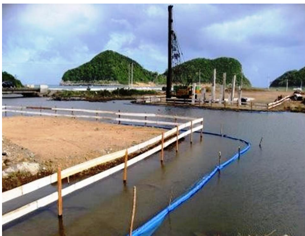
Measures were taken to mitigate the impact of the road construction on the environment. Curtains were installed at bridge and culvert sites to prevent sedimentation into the waterways. A wetland was created at the base of a high embankment area by planting Nypah palms, Giant leather ferns, Phragmites (reeds) and floating native species.
