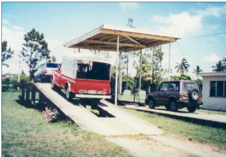
Plate 1: Simple low cost inspection ramp in Fiji.
