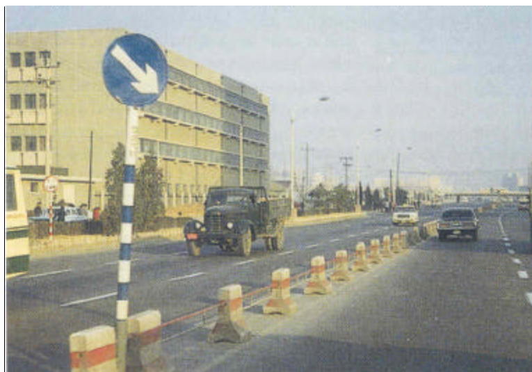
Plate 4 (above): Movable concrete block and steel rail barrier in the People's Republic of China (PRC).
