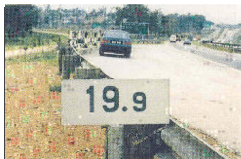
Plate 1: 100 m marker posts on an expressway in Malaysia.
