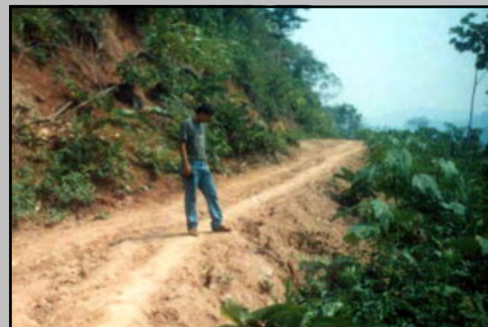
Unsurfaced rural road, San Martin Department (DVA 2006)
