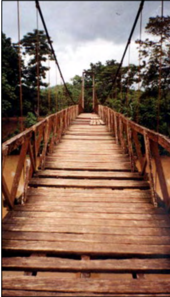
Footbridge over river GVA (2005)
