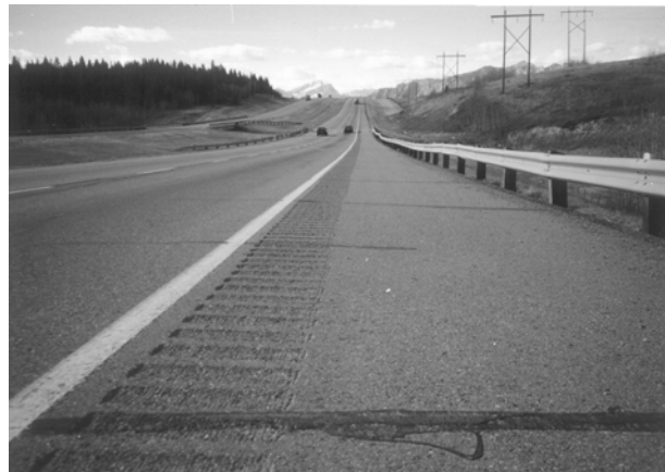
Figure 13. Divided highway with adequate recovery area, wide shoulders, no rigid obstructions and guard rails.
