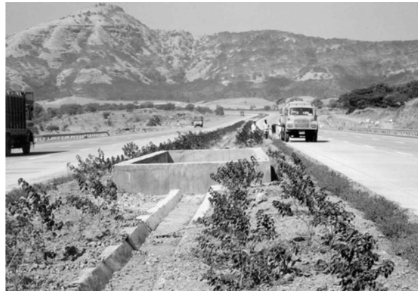
Figure 12. Rigid obstructions and high medians can be hazardous for high speed vehicle traffic
