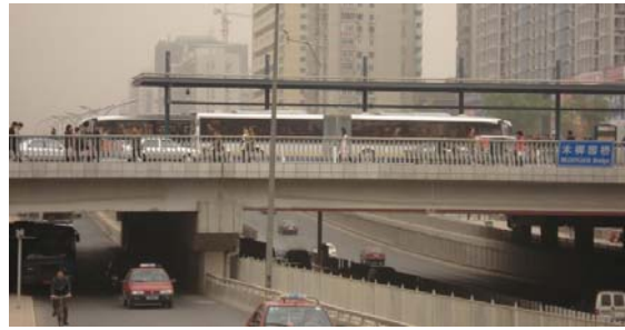
Beijing BRT Line 1 Station at Arterial Overpass
