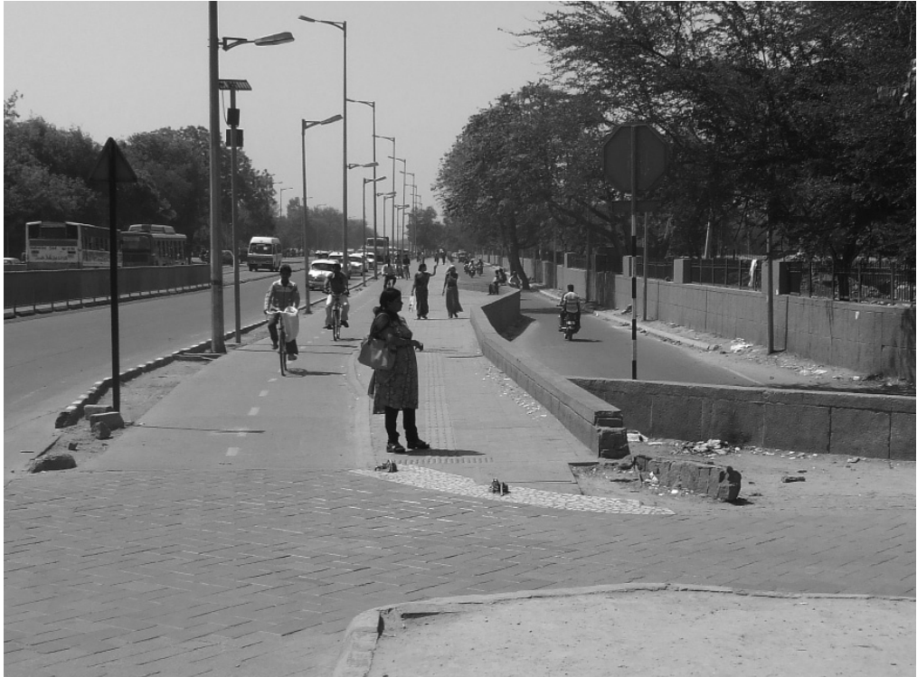
BRT corridor: Continuous sidewalks. Even access for vehicular passage does not interrupt
